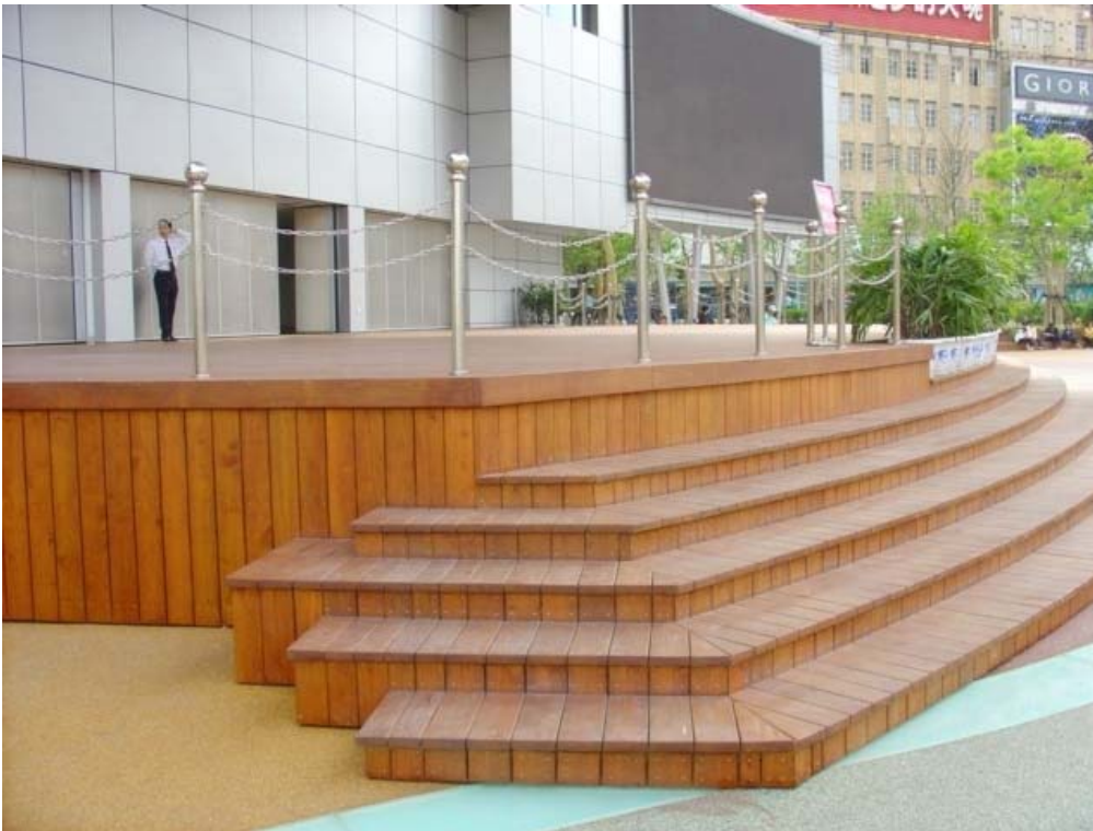
Photo 4: The project architect for the government-sponsored Century Square renovation project in downtown Shanghai selected US SYP for its beauty and ability to withstand heavy use.
