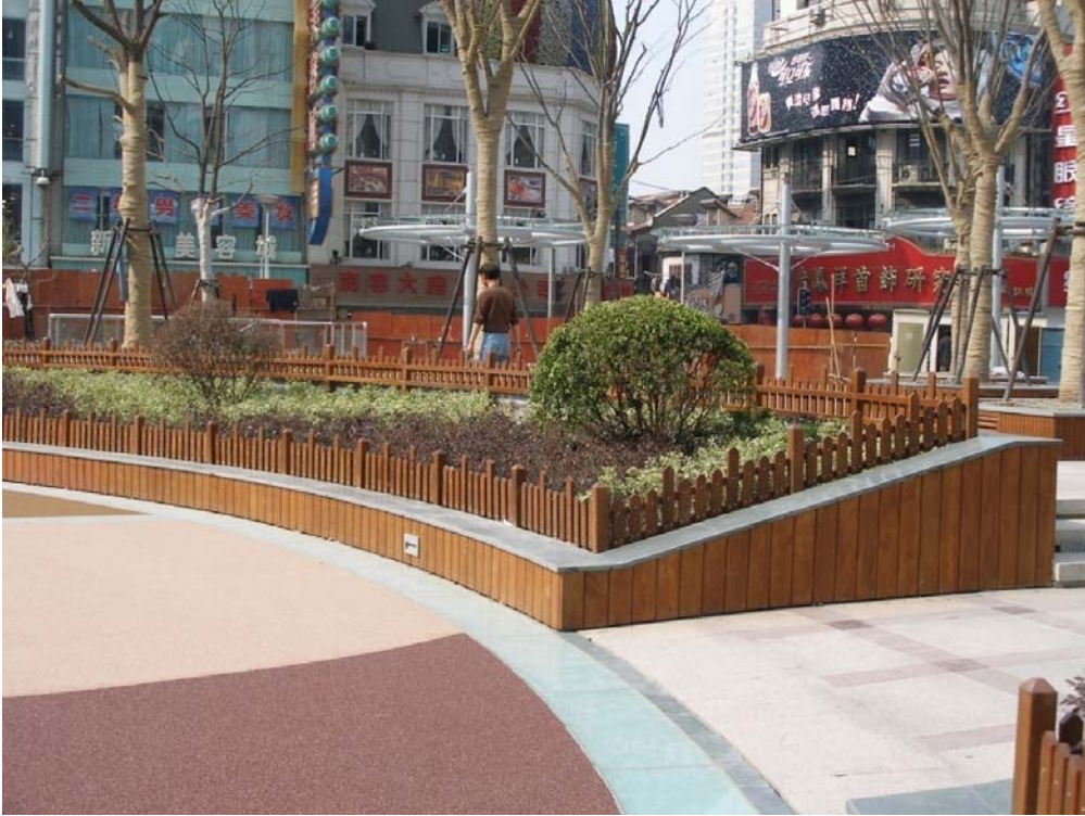
Photo 3: Southern yellow pine was used to build planters and as edging at the Century Square project at Shanghai's busy Nanjing Road shopping area.
