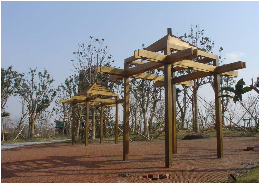
Photo 2: Local timber distributor, Xuelihua Timber Structure Engineering Company, supplied SYP for the Holland New City development, provided technical advice, and helped the project designer reduce waste by modifying designs to fit US lumber dimensions.
