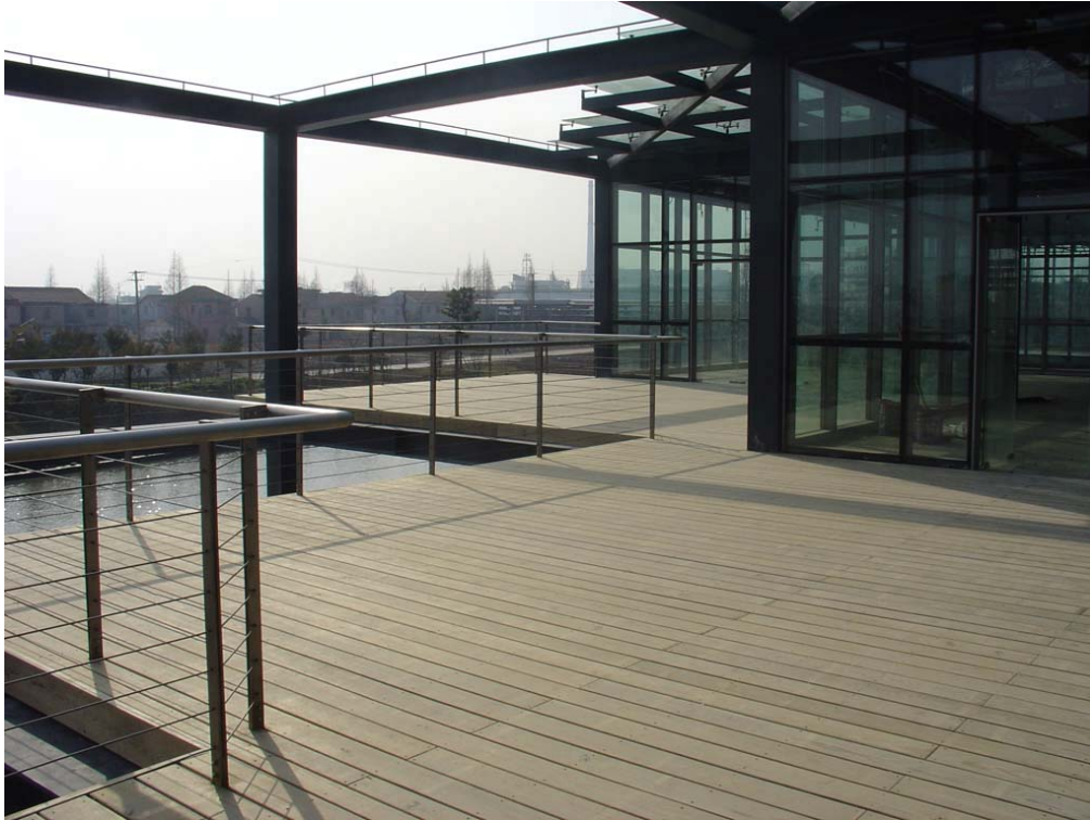
Photo 1: Southern yellow pine was used to build the deck at the sales office for the Holland New City project in Pudong, a suburb of Shanghai. After the project is sold the sales office will become a clubhouse.
