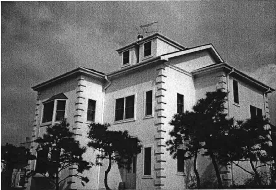
Figure 19. Stucco finish on high-end wood frame home in Ilsan.
