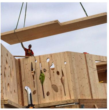
Figure 2. Cross Laminated Timber CLT used in building (Source: forterrs.org; photo credit: atelier jones)
