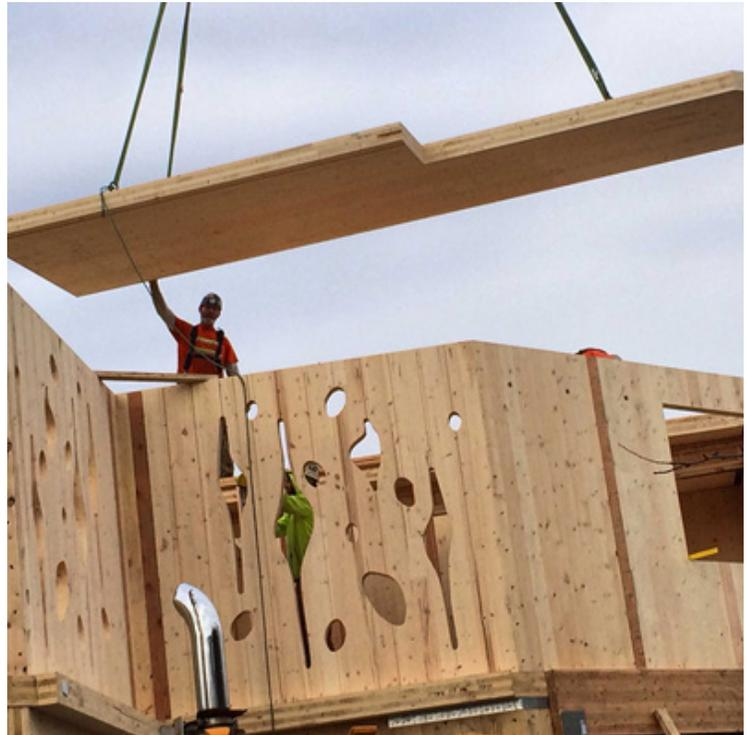
**Figure 2. Cross Laminated Timber CLT used in building**
